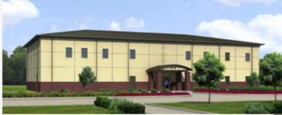
3-81 AR Company Operations Facility
